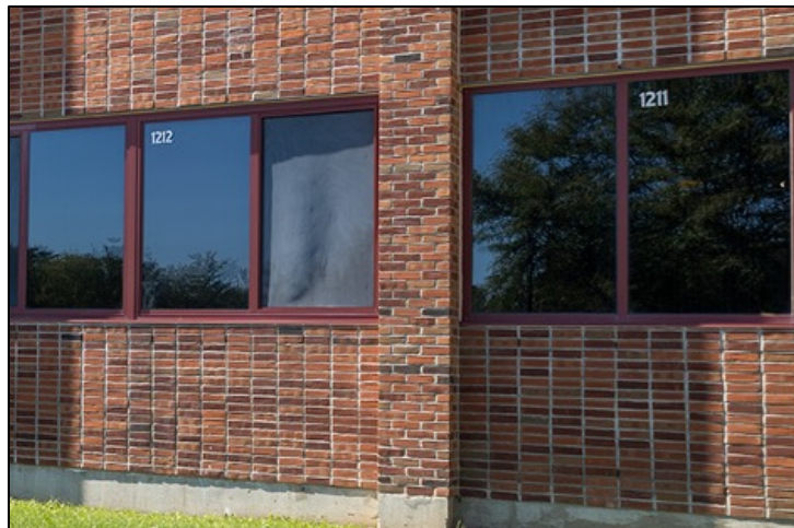
Figure 2: Reflective glazing film
