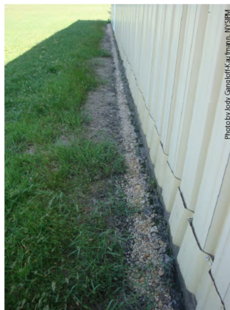
Simple modifications, like this gravel barrier around the building, can reduce pest activity inside.
