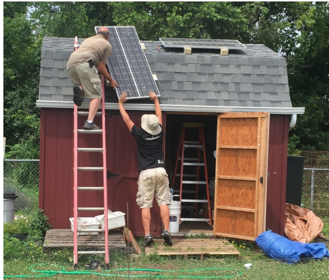
Solar panel installation on a shed in the Big Hill Farm student garden
